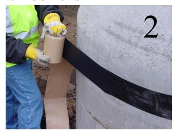
2. Remove the first foot of paper backing from the mastic. Center and place the Gator Wrap® around the joint. Continue to remove paper backing as you apply the Gator Wrap to the entire structure.
