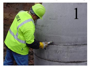
1. Expose the area that is to be sealed. Clean the entire area around the joint with a wire brush and whisk broom. Remove any sharp protruding edges around the joint with an abrasive tool. When finished cleaning, the entire area must be dry and free of any dirt.
